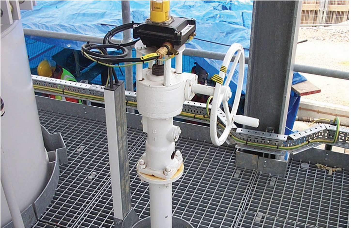
GENERAL VALVE Twin Seal plug valve fitted with enclosed limit switches.
